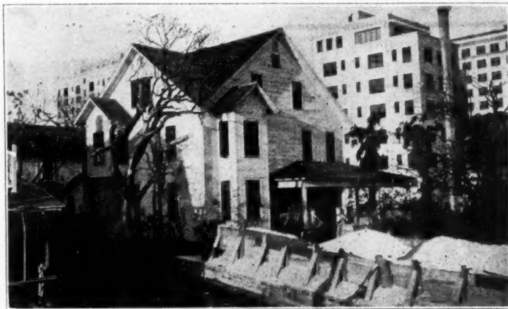
Left—This frame house of E. W. Crane, Hallendale, sheltered 10 neighbors, 110 chickens, three dogs and a cat during the storm and came through without damage. It is sixteen feet square at the base and fourteen feet square at the fourth floor. Mr. Crane lived formerly in North Dakota and built his house to stand. Right—The Alhambra, a small boarding house in Miami. The only damage was caused by water. The wood shingle roof is in perfect condition although laid fifteen years ago. Seven boats and barges were driven into the yard by wind and waves.
